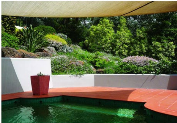
Rendered tanks used as a retaining wall and garden bed
