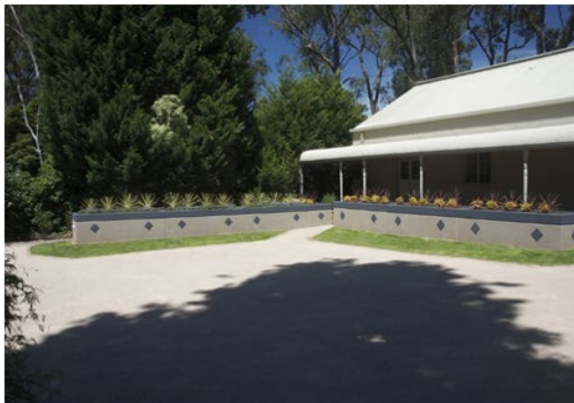
Tanks used as a boundary and garden bed
