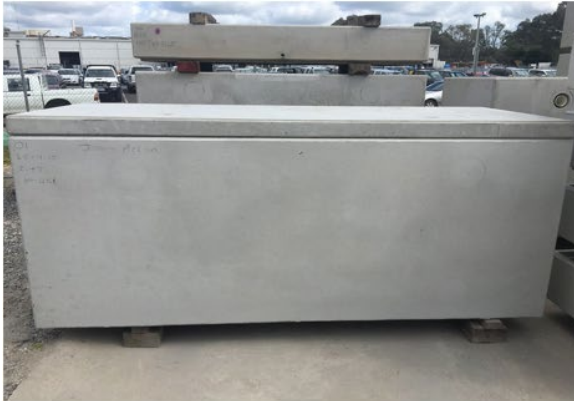
A finished raw concrete tank
